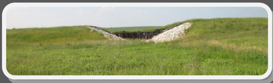
WELL MAINTAINED STRUCTURE
