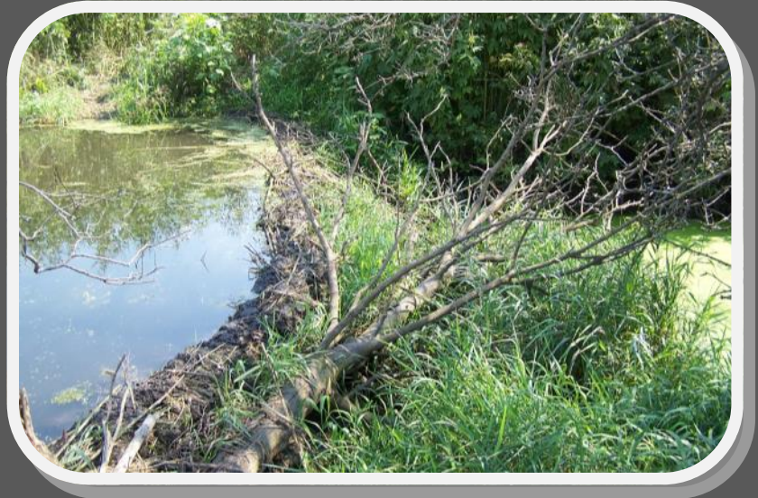
BEAVER DAM RAISES AT THE INLET TO THE WETLAND. COULD RAISE THE WATER LEVEL WHICH COULD INUNDATE INCOMING TILE OUTLETS
